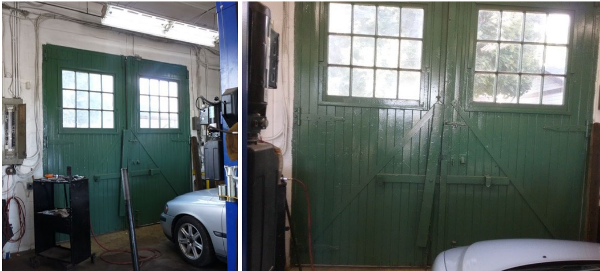
Interior of the wood doors, photographed in September 2016
