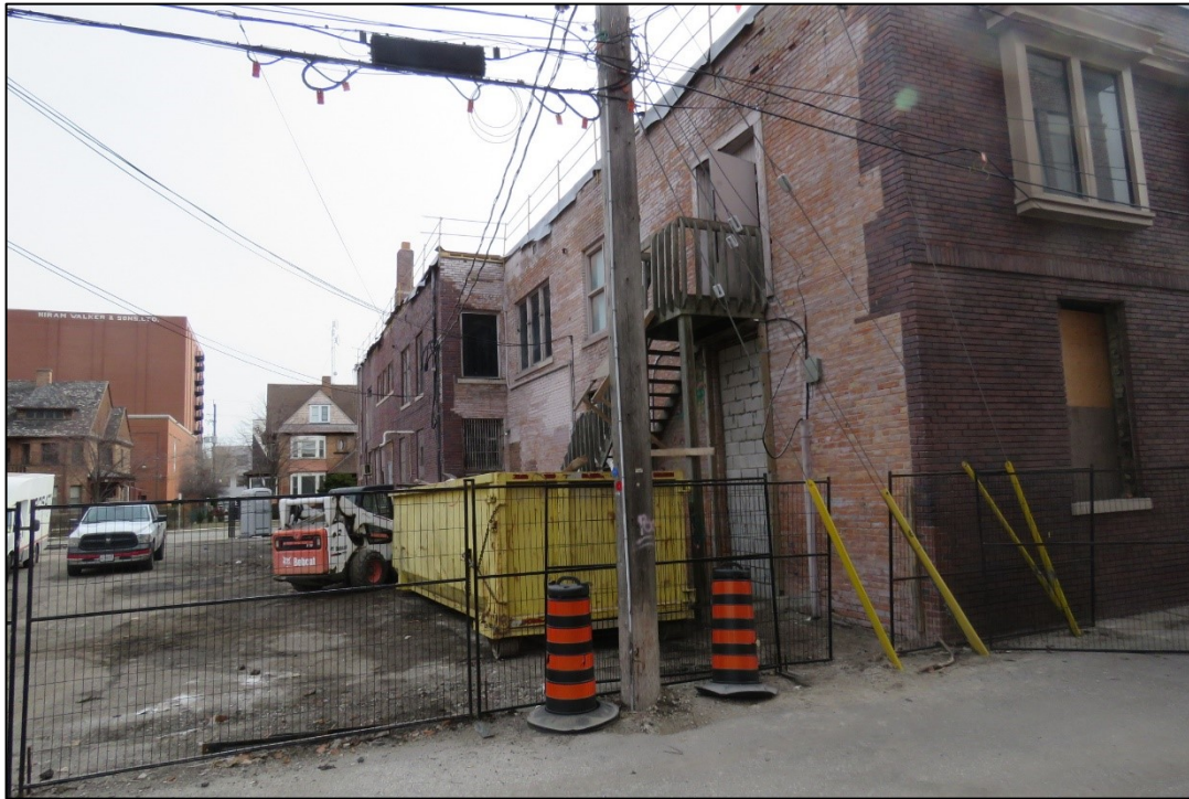
Figure 7 - Rear of 1958-1998 Wyandotte Street East, looking east from subject alley
