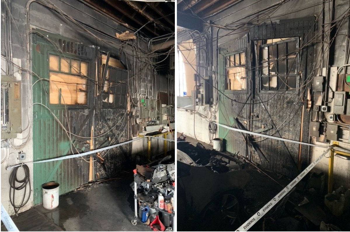
Interior of the wood doors immediately following the work shop fire, photographed by owner in January 2022
