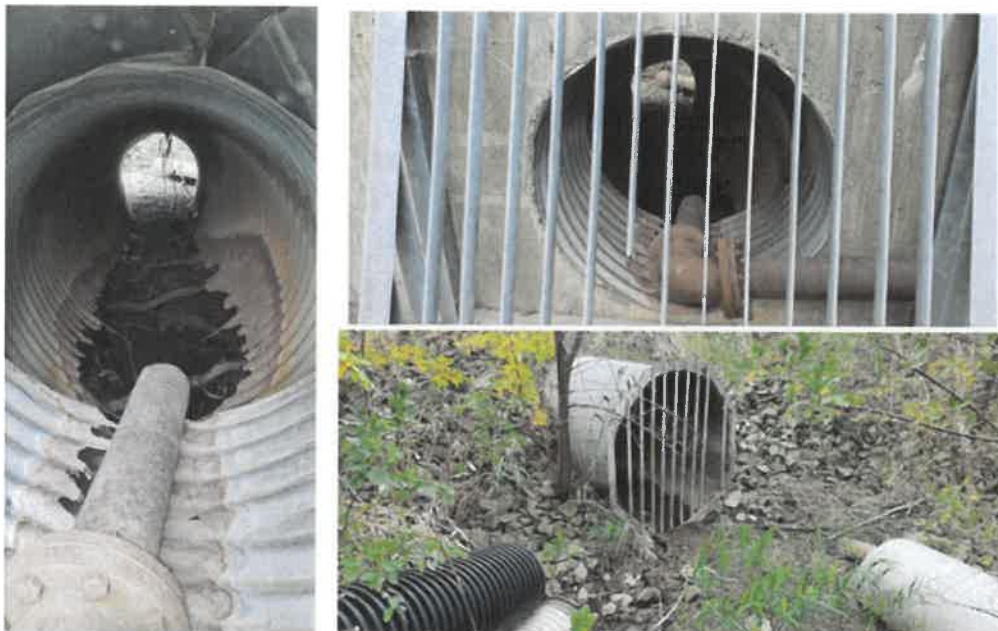
Photograph #2 – Current Central Pond Outlet
