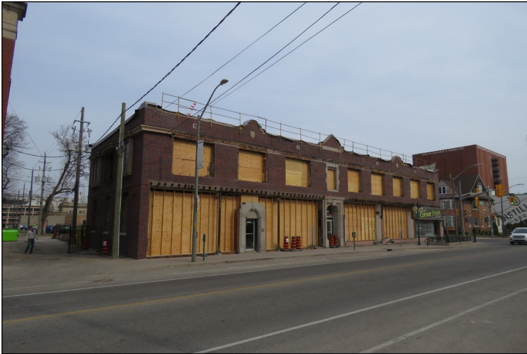
Figure 11 - Front of 1958-1998 Wyandotte Street East, looking north from Wyandotte Street East
