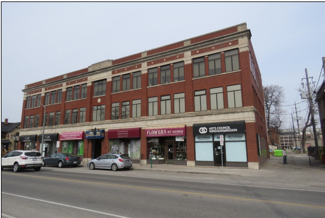
Figure 12 - Front of 1900-1942 Wyandotte Street East, looking north from Wyandotte Street East
